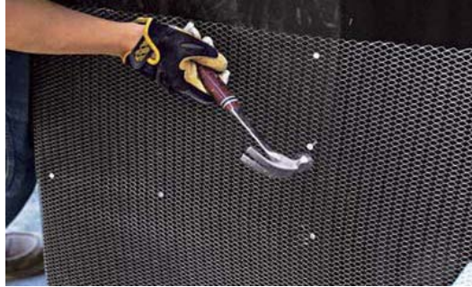
Figure 4.6, Wall Lath for Stucco
